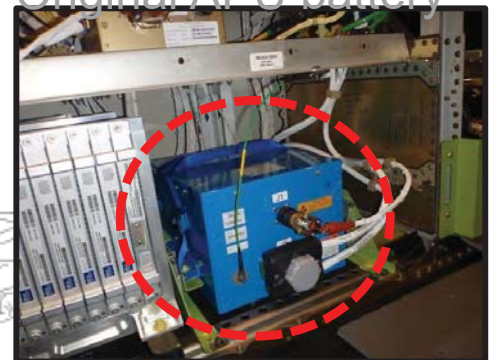
Original APU battery
